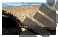
Asbestos is the generic term for a number of fibrous silicate minerals. Products made from asbestos cement – a bonded asbestos material – include fibro sheeting (flat and profiled) guttering and downpipes, as well as other pipes for water, drainage or flues, corrugated roofing sheets, roofing shingles and guttering.
