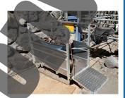
A materials hoist is a type of builder's hoist with which goods or materials may be raised or lowered. Workers are **NOT** allowed to ride in a materials hoist.
