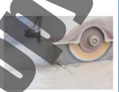
When the concrete does shrink and crack, the control joint is placed so that the slab will crack on a line instead of randomly across the slab.
