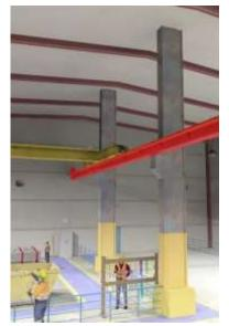
When the carriage travels the length of an area it is called **long travelling**. For this a crane needs a **runway**.
